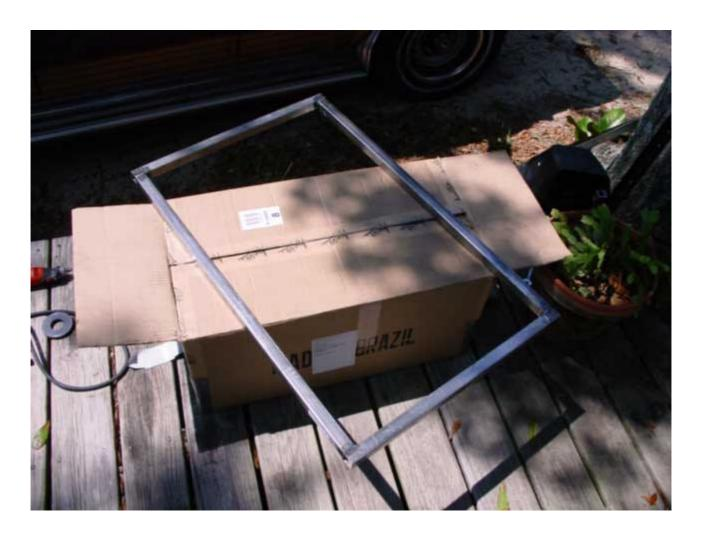
Once the cut work is done, two of the 31 3/4" lengths and two of the 21 3/8" lengths are welded to form a rectangle. This is repeated to form the second. These will be the front and back openings and rack rail support struts for the rack cabinet's frame. Welding magnets make this process easy, by holding the tubing in place and keeping the angle 90 degrees.
